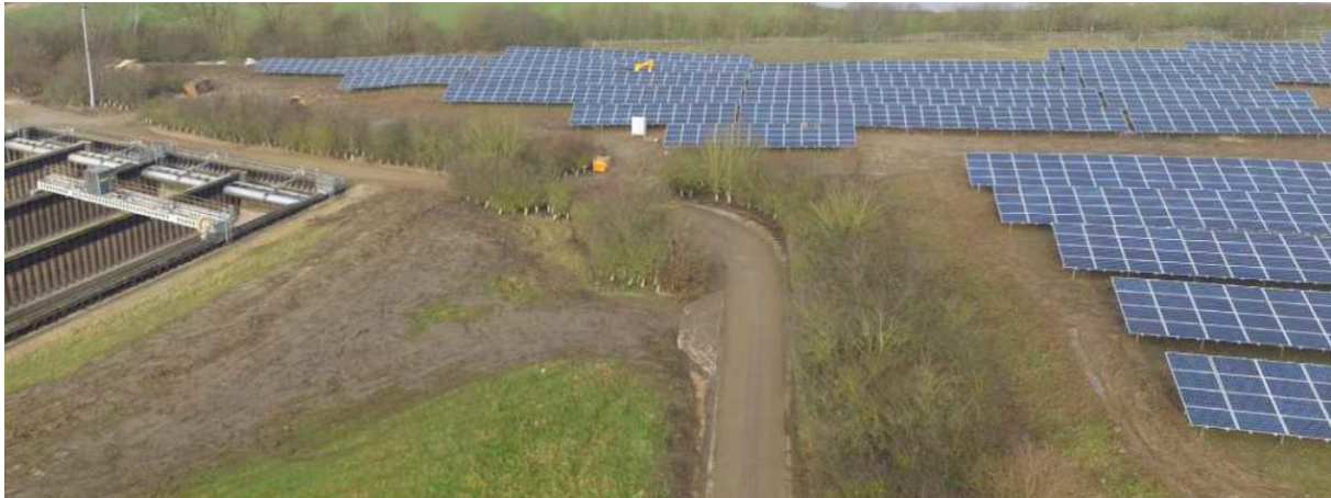
Figure 11 Installation of solar panels at one of Anglian Water 's operational sites
