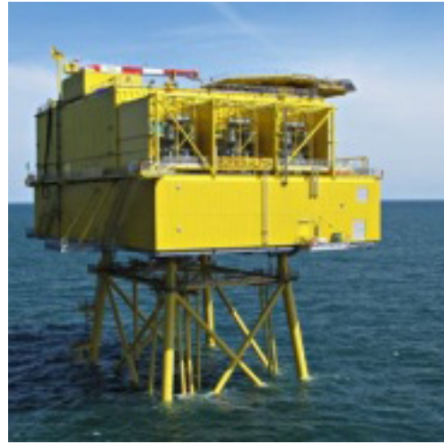
5b. Borwin Alpha, VSC HVSC converter station
