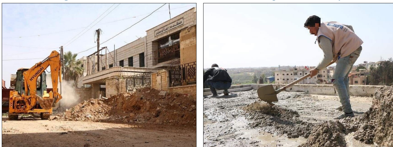
Figure 1. Reconstruction Works at the National Hospital, Daraa City
