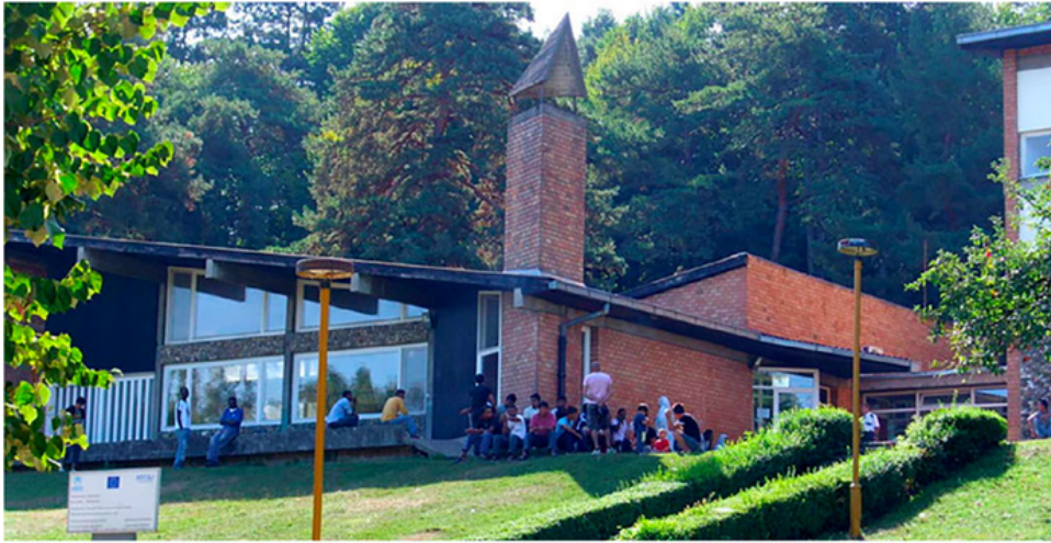
Present-day appearance of the United Nations Refugee centre in Banja Koviljača, designed by Architect Mihajlo Mitrović and built in 1964 (Staničić 2022, 184).
