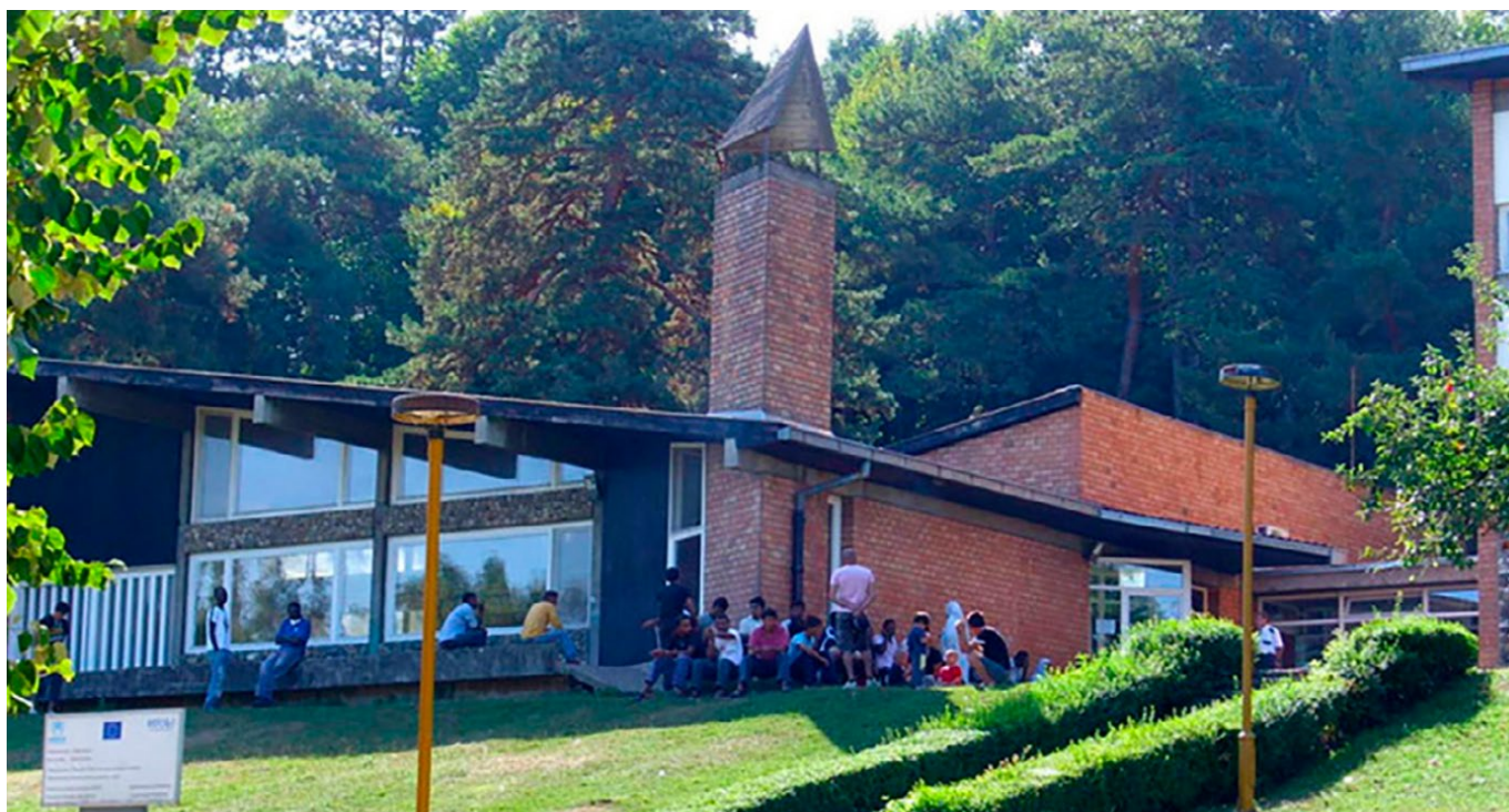
Present-day appearance of the United Nations Refugee centre in Banja Koviljača, designed by Architect Mihajlo Mitrović and built in 1964.
